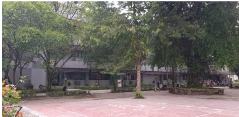
Fig.3. the Side View of J14 Building
