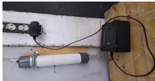
Figure 6. Device Connected to an electrical outlet
